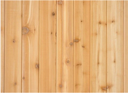
Sauna Area Ceiling & Walls: Knotty Finesline Cedar w/ Clear Sealer
