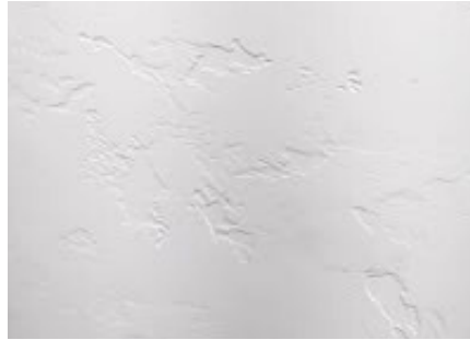
Fit/Plunge Area Ceiling & Walls: Hand Textured Walls
