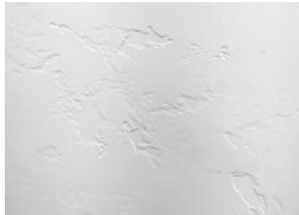
Fit/Plunge Area Ceiling & Walls: Hand Textured Walls
